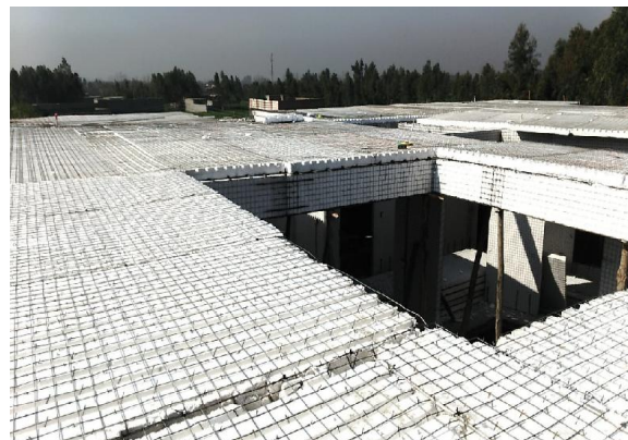
Figure 06: Placed Slab panels on wall panels
