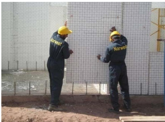
Figure 05 : Placing panels in dowels
