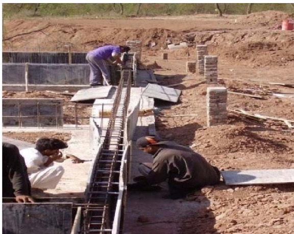
Figure 02: Making of foundation
