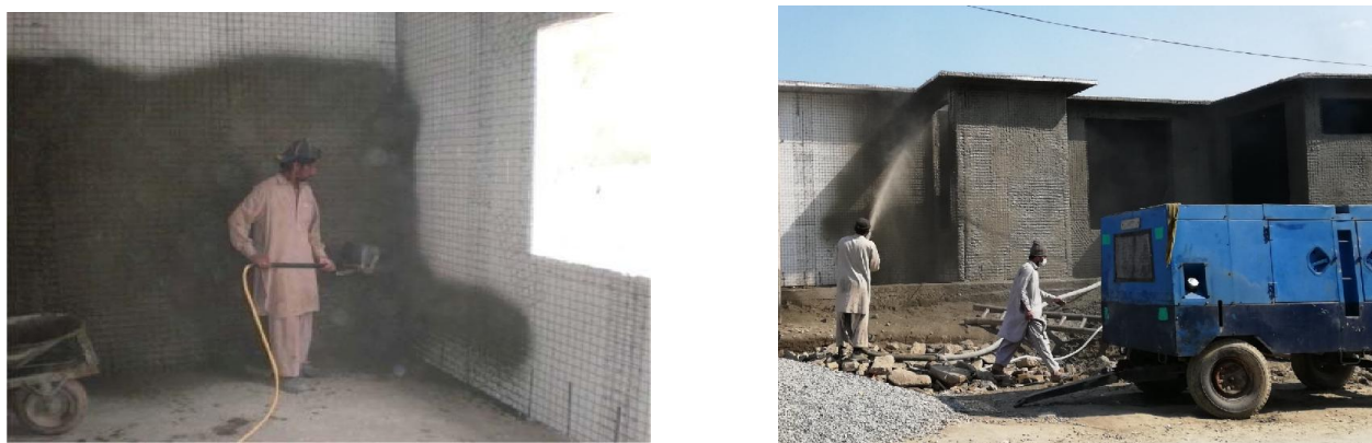
Figure 08:Applying Concrete
