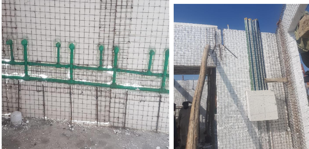
Figure 07: Installation of utilities before concretion
